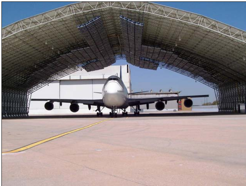
Figure 7-7. Infrared Hangar at JFK
