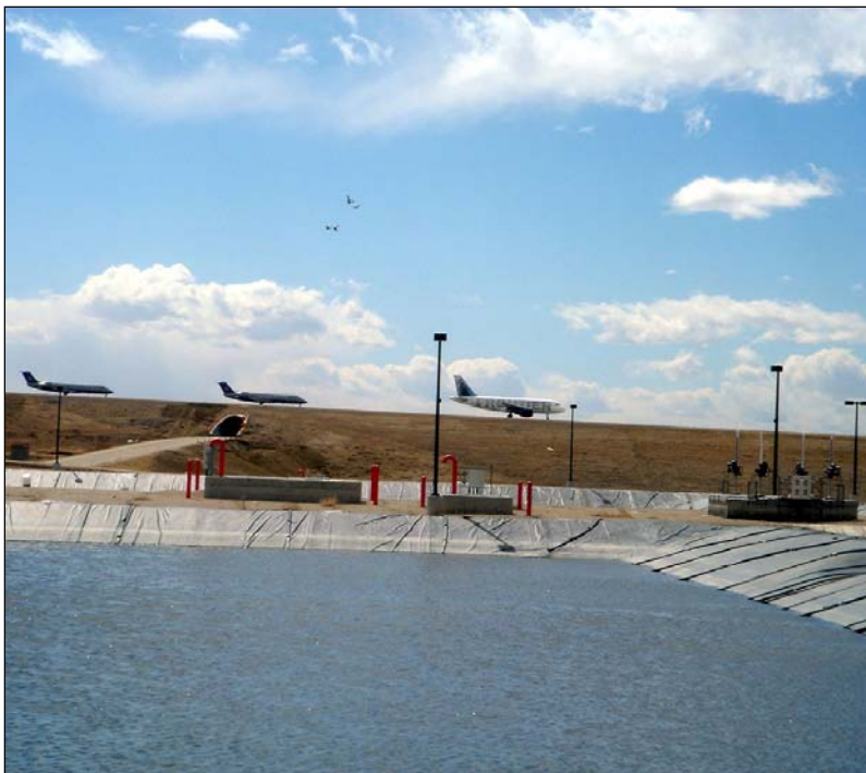
Figure 7-3. Pond for Deicing Stormwater Storage
