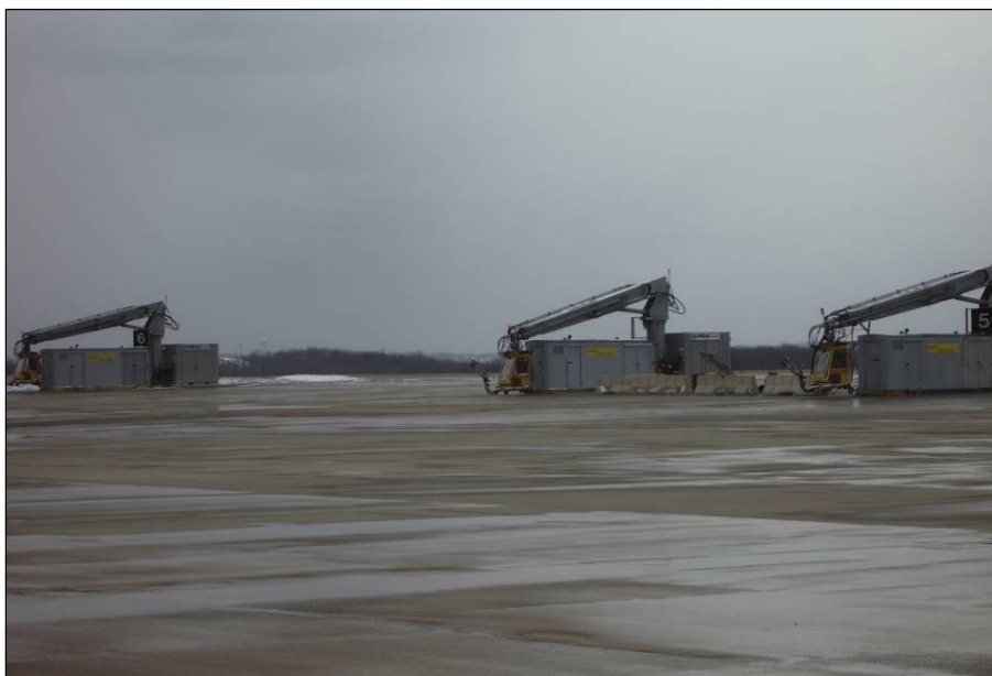
Figure 7-1. Deicing Pad Equipped with Fixed Deicing Booms at Pittsburgh Airport
