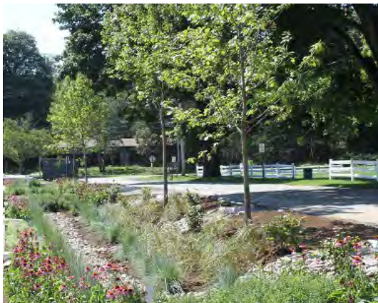
Bioswales and raingardens as filtration systems
