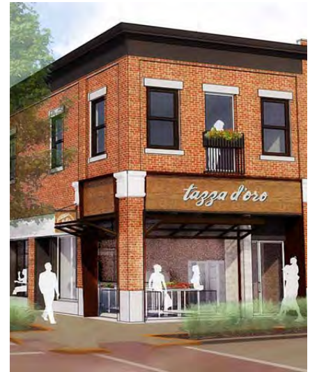
Example of a retail building designed to accommodate some flooding on the ground floor using garage door-style openings at the lowest elevation, tile and concrete floors and walls, and elevating equipment above the floodplain.
