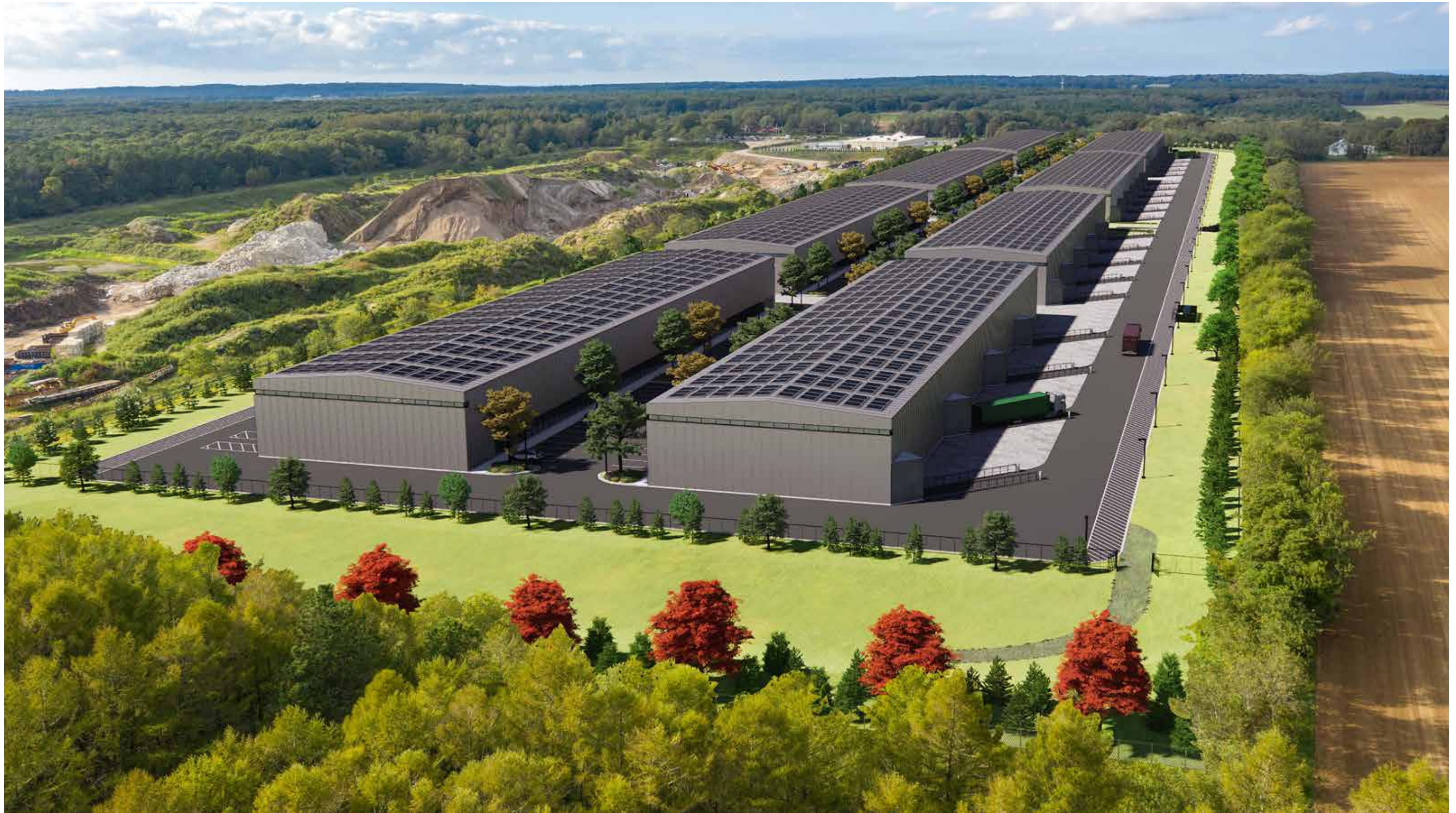
VIEW 5 - SOUTH AERIAL
