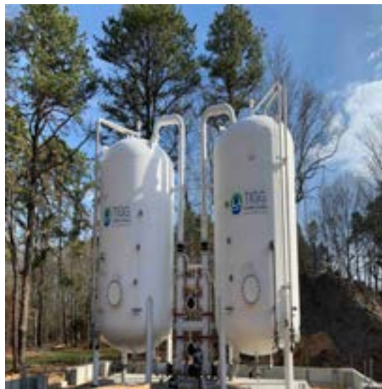
GAC filters used for removal of PFA compounds
