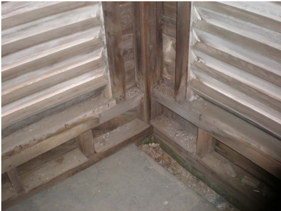
INTERIOR BASE AND SILL AT LOUVERS
