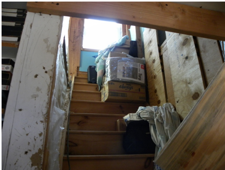
Photo 10: interior staircase leading to added third story “tower”
