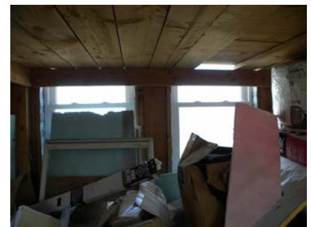
Photo 16: interior of third floor tower
