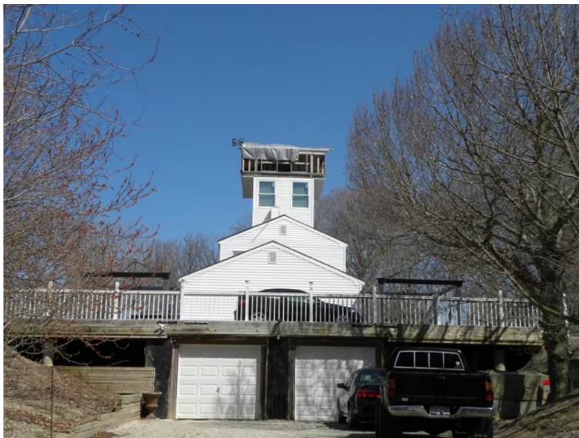
Photo 1: west elevation of subject structure
