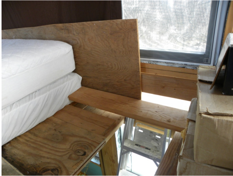
Photo 22: construction floor dividing third story tower. Access is by ladder and small opening looking down into lower level of third story tower.
