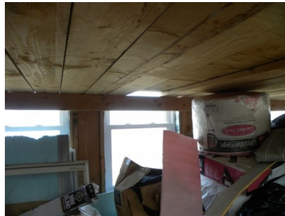
Photo 18: interior of third floor tower
