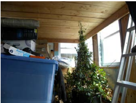
Photo 14: interior of third floor tower
