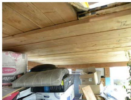
Photo 15: interior of third floor tower Note plank construction floor overhead
