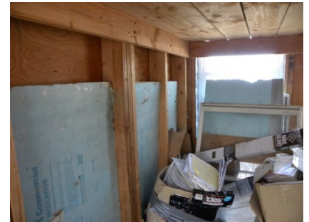
Photo 19: interior of third floor tower
