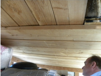
Photo 17: interior of third floor tower Note plank construction floor overhead
