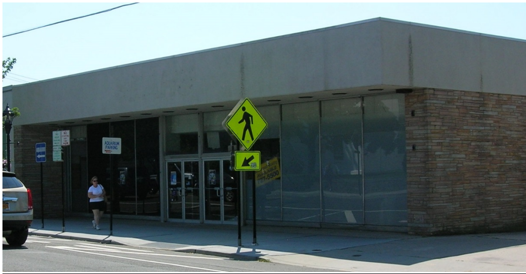
The former Sears Department store has been closed since 2006. The building will be sold in 2016 to a new owner.
